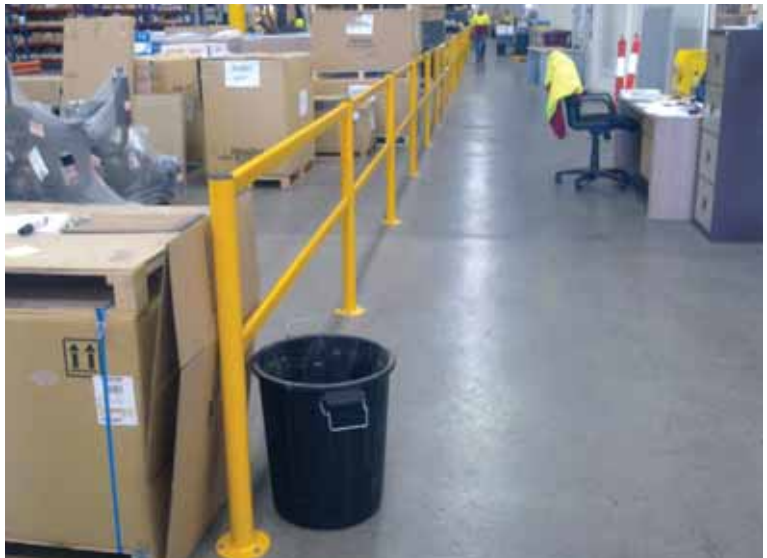
All rails and posts are galvanised and powder coated.
